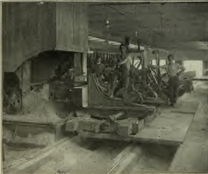
FIG. 3. RIGHT-HAND BAND MILL DRIVEN BY 150-HORSEPOWER MOTOR
